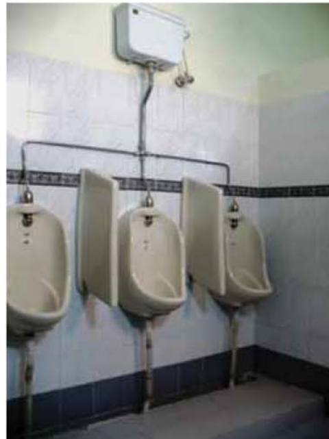
Figure 2.11b: Auto Flushing Tank
