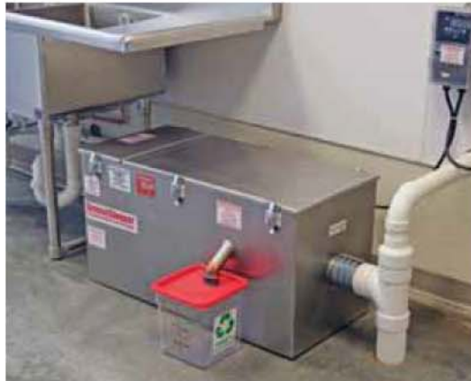
Figure 2.13b: Grease Interceptor–Installed
