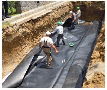
Installation of the geomembrane on top of the protection geotextile Photos during the construction and installation
