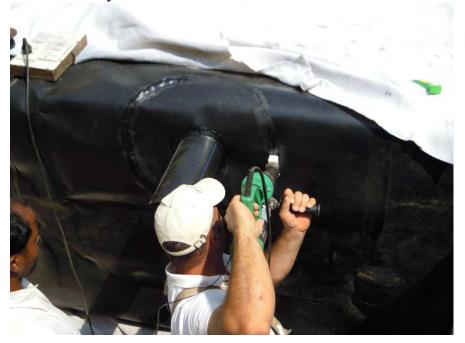
Detail of the connection, covering with the geomembrane
