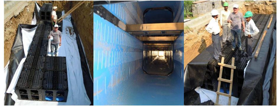
End of the box installation and covering of the basin with the geosynthetics
