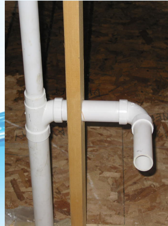
Kitchen Sink Rough In – 40 mm Trap Arm to 50 mm Drain
