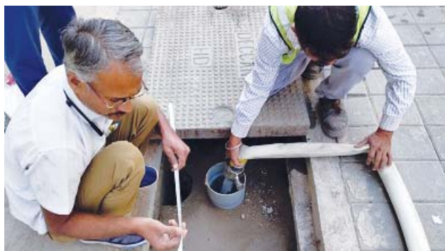
Water being poured in the borewell to test its recharge capacity
