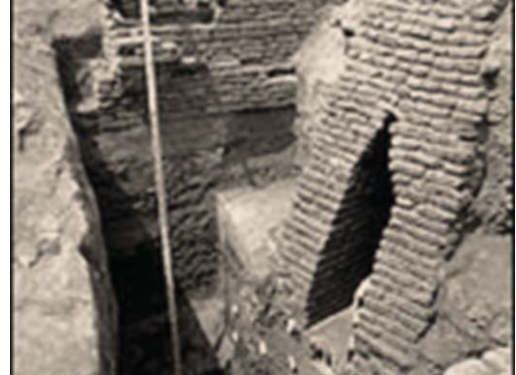
This large corbelled drain was built in the middle of an abandoned gateway at Harappa to dispose of rainwater and sewage.
