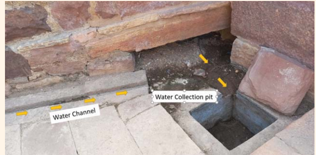
Fig. 6: Water collection system
