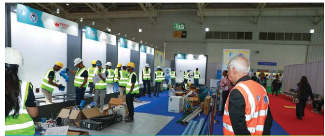
Participants in process of making the bathroom under jury supervision
