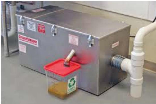
Fig 2: Under sink grease interceptor (for small kitchens)
